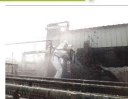
洩漏點初步止漏
