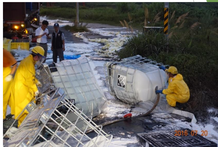
嚴重變形TANK只好現地抽除移槽
